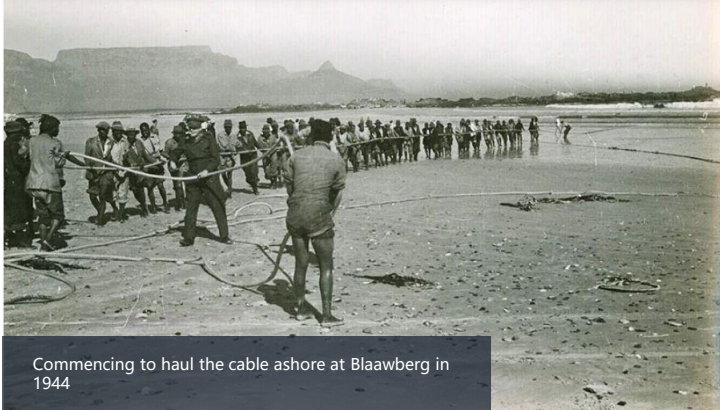
Laying an undersea cable in Cape Town
